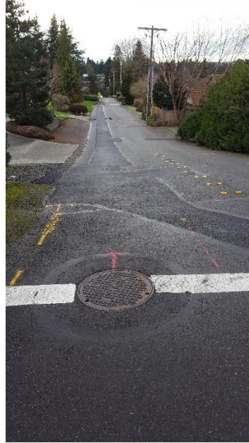
CB 1113 (Looking West)
