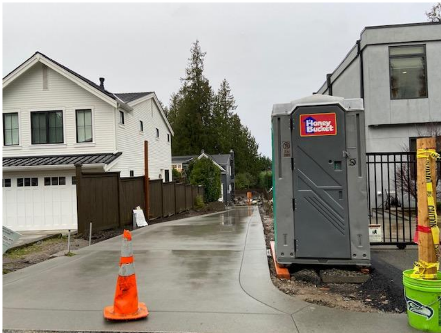
Example of on site parking violation on 94 th Ave N.E., construction vehicles are parked on the street
