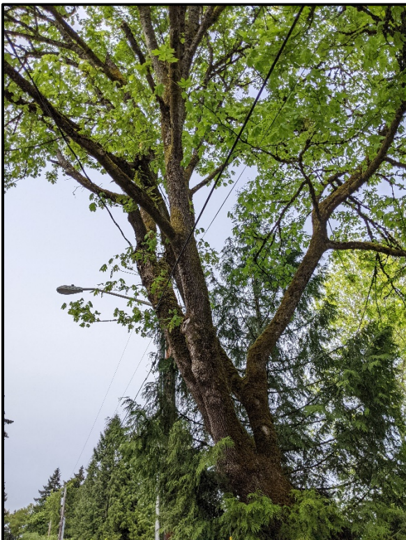
Photo 2. Power lines running along east side of 95 th Ave NE in contact with tree in some places.
