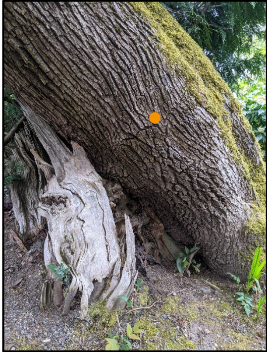
Photo 6. Looking north at south side of tree base; orange dot indicates location of drill test 2.
