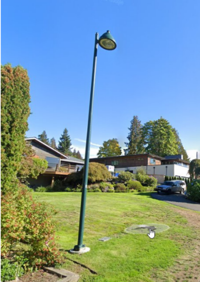
4408 92 nd Ave NE – Typical 25-ft tall street light
