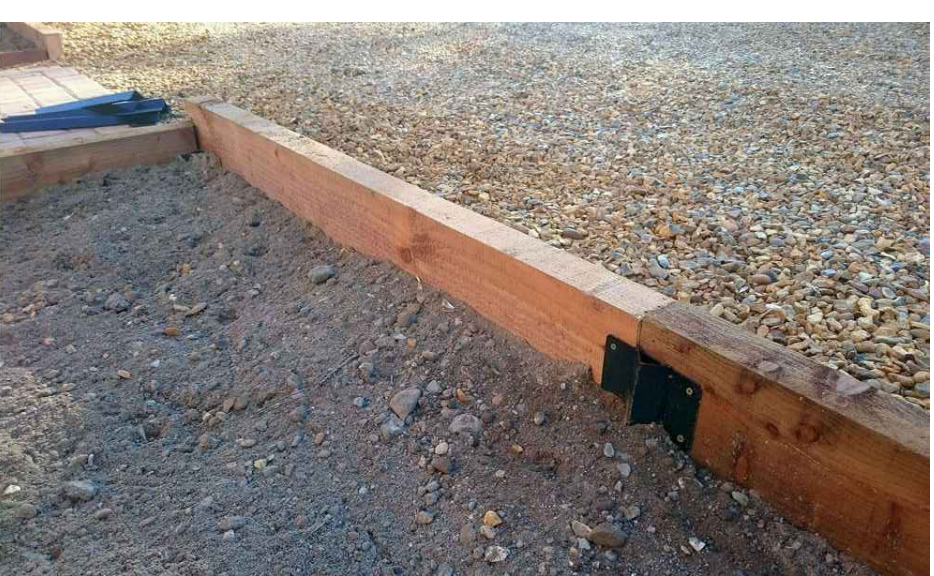
B TIMBER CURB AT DRIVEWAY
