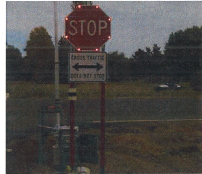
Flashing LEDs around stop sign face (MnDOT).
