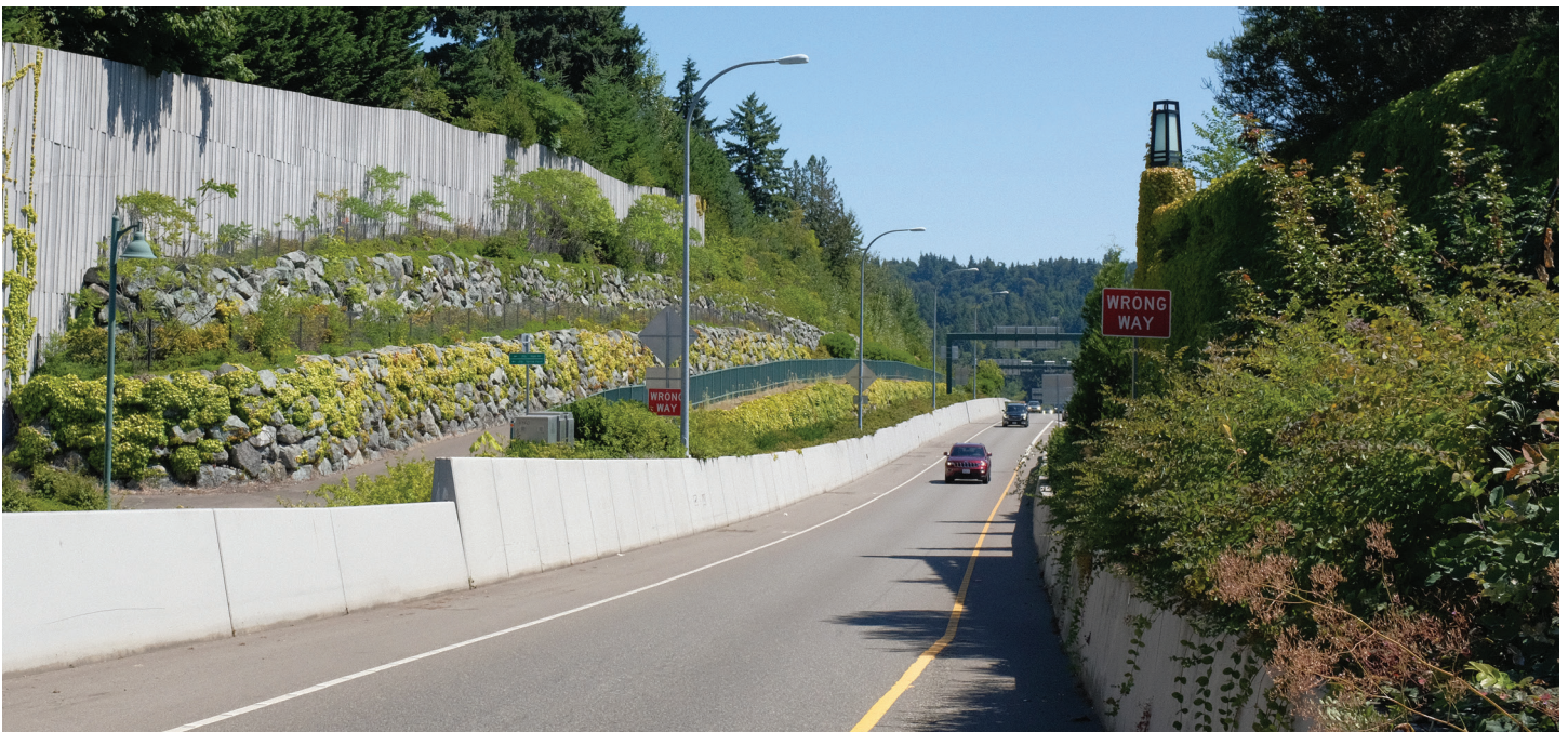
Figure 55. Ramp onto SR-520 (Smith, 2023)
