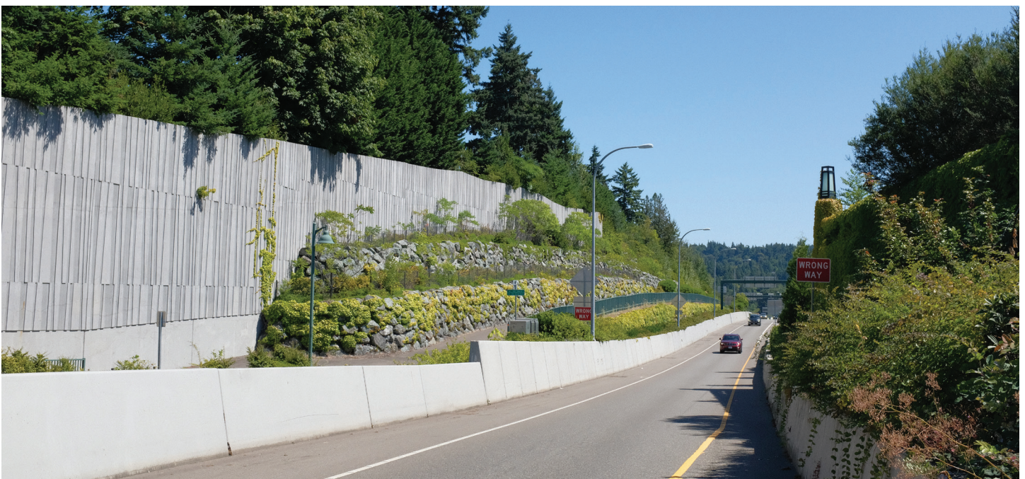
Figure 46. Ramp onto SR-520 (Smith, 2023)
