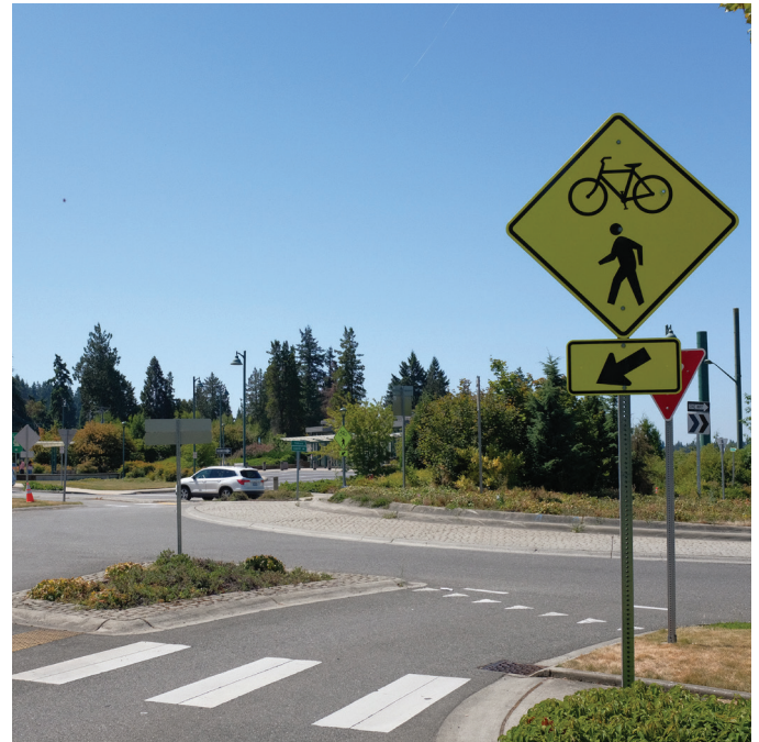
Figure 32. Yarrow Point Road Roundabout (Smith, 2023)
