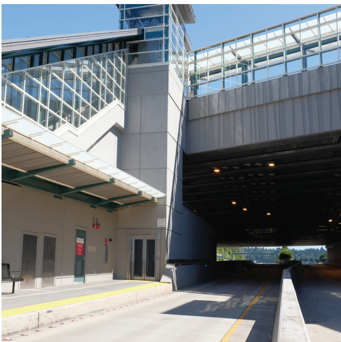
Figure 35. King County Metro Infrastructure (Smith, 2023)
