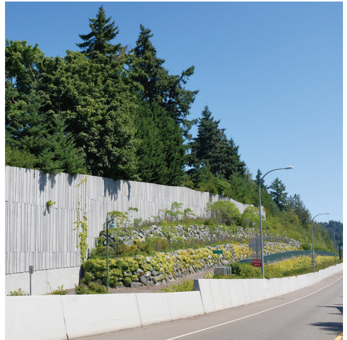
Figure 41. Ramp Barrier Toward SR-520 (Smith, 2023)
