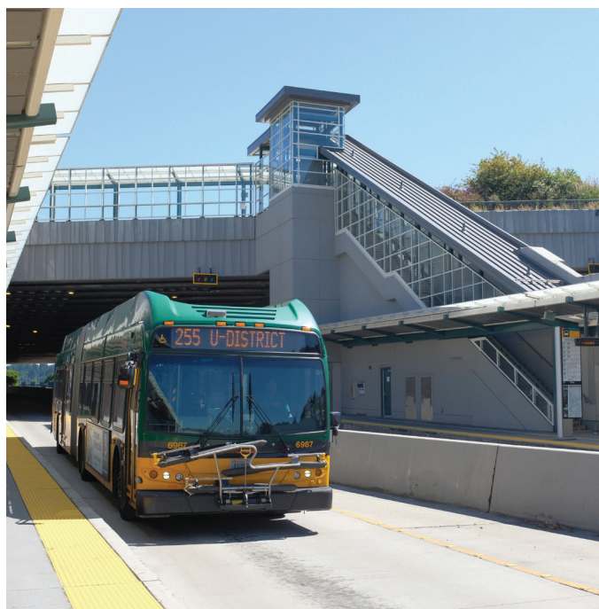
Figure 34. King County Metro Infrastructure (Smith, 2023)
