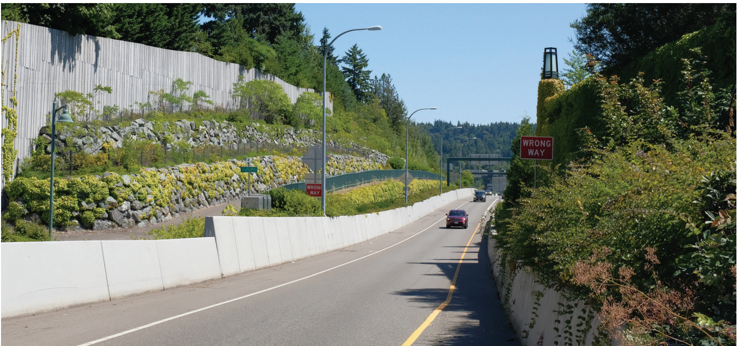
Figure 55. Ramp onto SR-520 (Smith, 2023)
