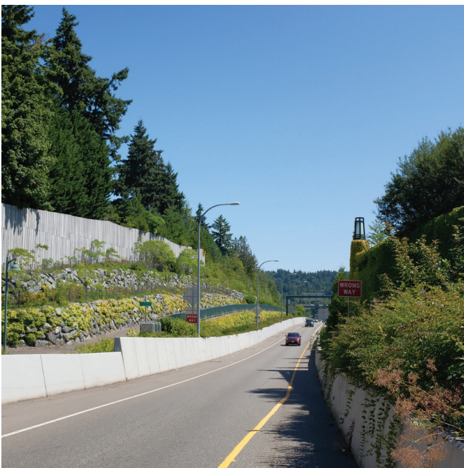
Figure 37. Freeway 520 Ramp (Smith, 2023)
