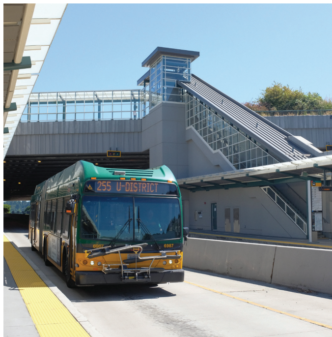
Figure 34. King County Metro Infrastructure (Smith, 2023)
