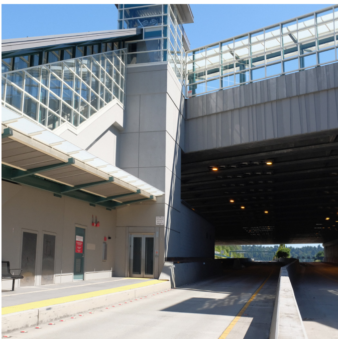
Figure 36. King County Metro Infrastructure (Smith, 2023)
