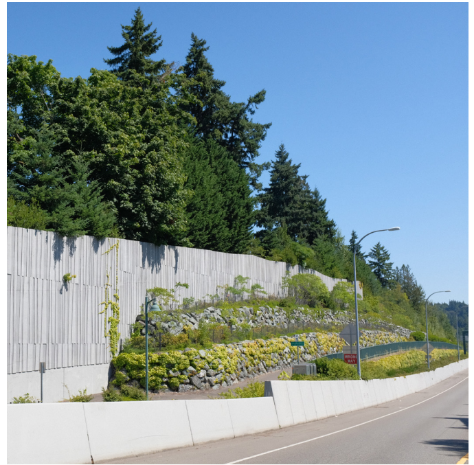
Figure 44. Ramp Barrier Toward SR-520 (Smith, 2023)
