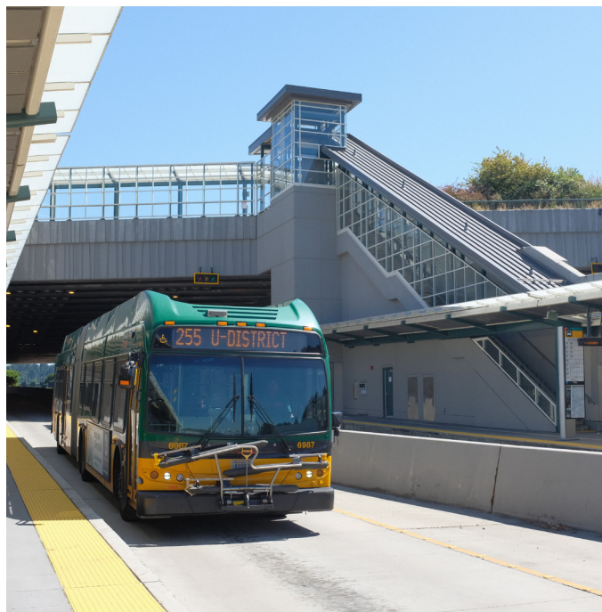
Figure 35. King County Metro Infrastructure (Smith, 2023)
