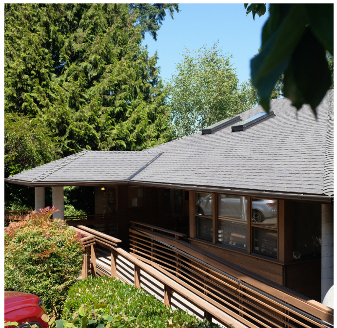
Figure 24. Yarrow Point Town Hall (Smith, 2023)
