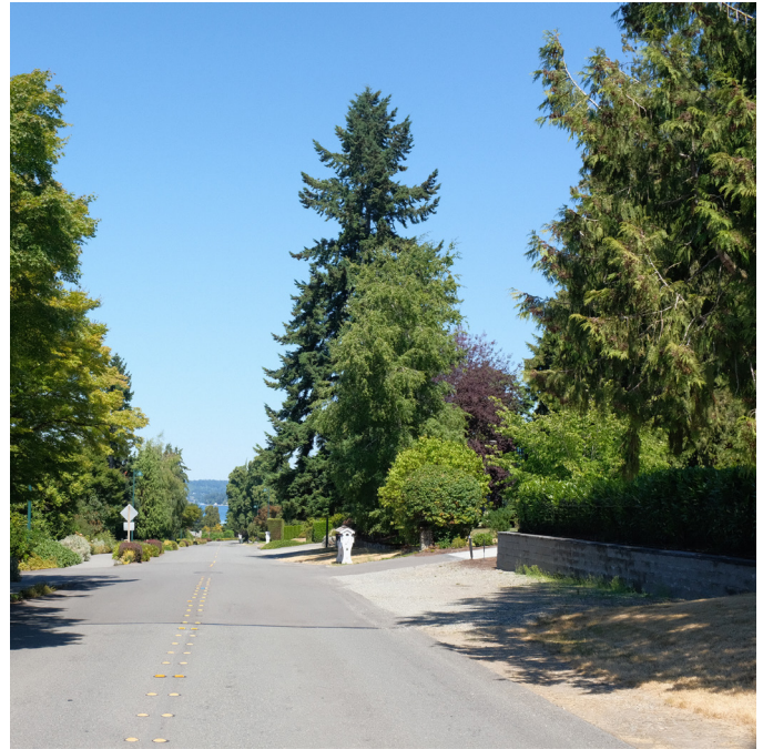
Figure 42. 94th Ave NE (Smith, 2023)
