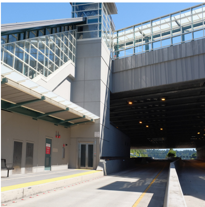
Figure 36. King County Metro Infrastructure (Smith, 2023)
