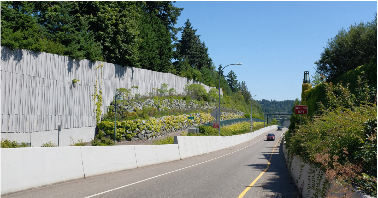
Figure 81. Ramp to SR-520 (Smith, 2023)
