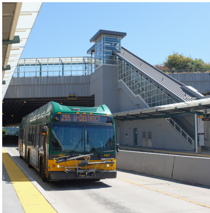
Figure 35. King County Metro Infrastructure (Smith, 2023)
