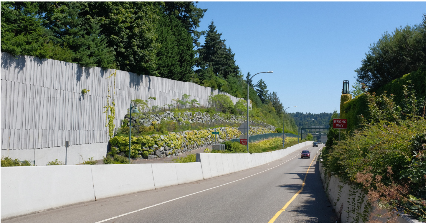
Figure 81. Ramp to SR-520 (Smith, 2023)
