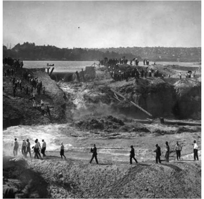
Figure 9. Montelake Cut (MOHAI, 1916)
