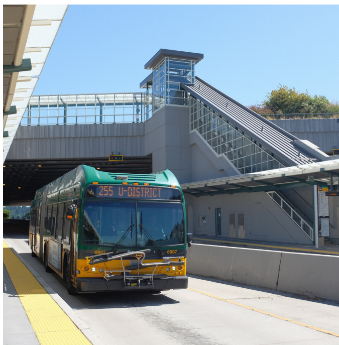
Figure 35. King County Metro Infrastructure (Smith, 2023)
