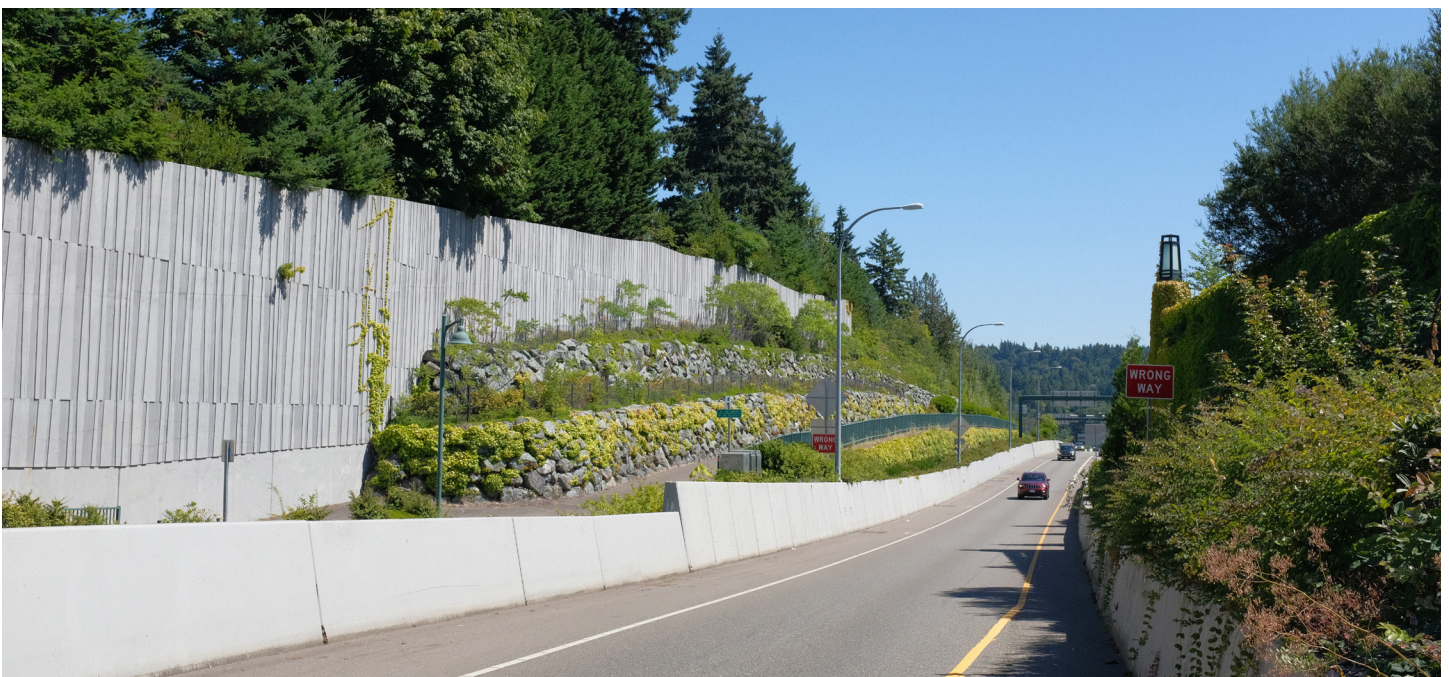
Figure 49. Ramp onto SR-520 (Smith, 2023)
