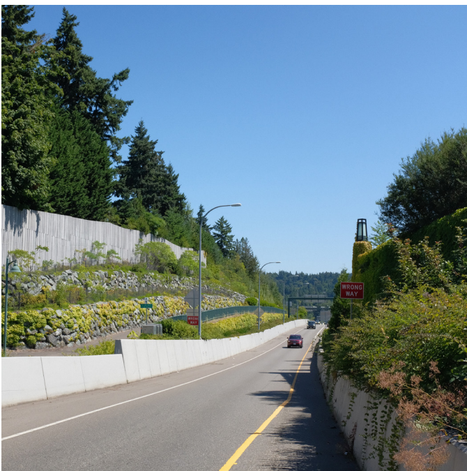
Figure 38. Freeway 520 Ramp (Smith, 2023)
