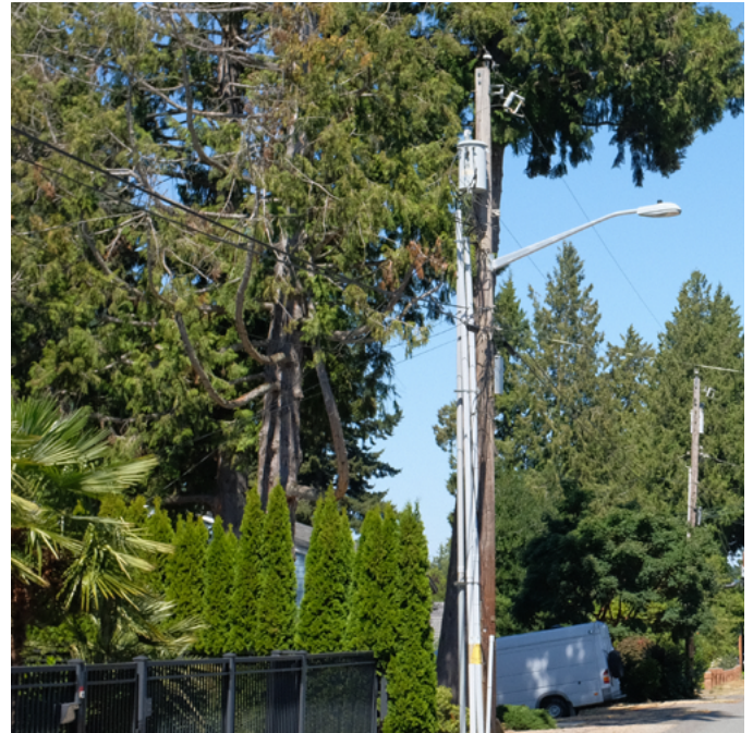
Figure 74. Utility Pole (Smith, 2023)
