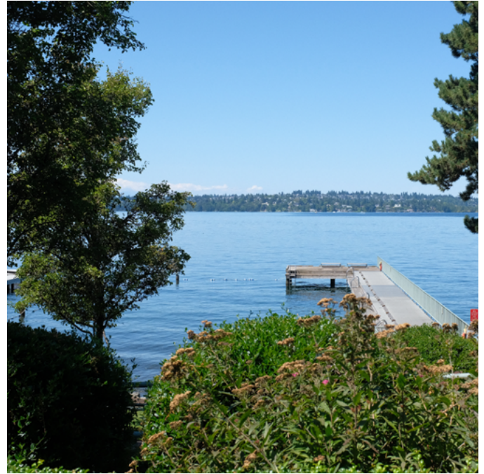
Figure 65. Road End Beach Pier (Smith, 2023)
