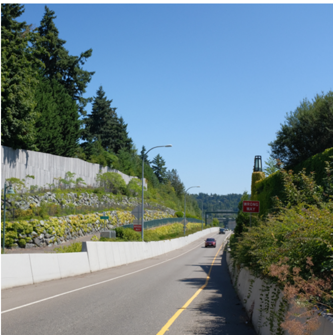
Figure 35. Freeway 520 Ramp (Smith, 2023)
