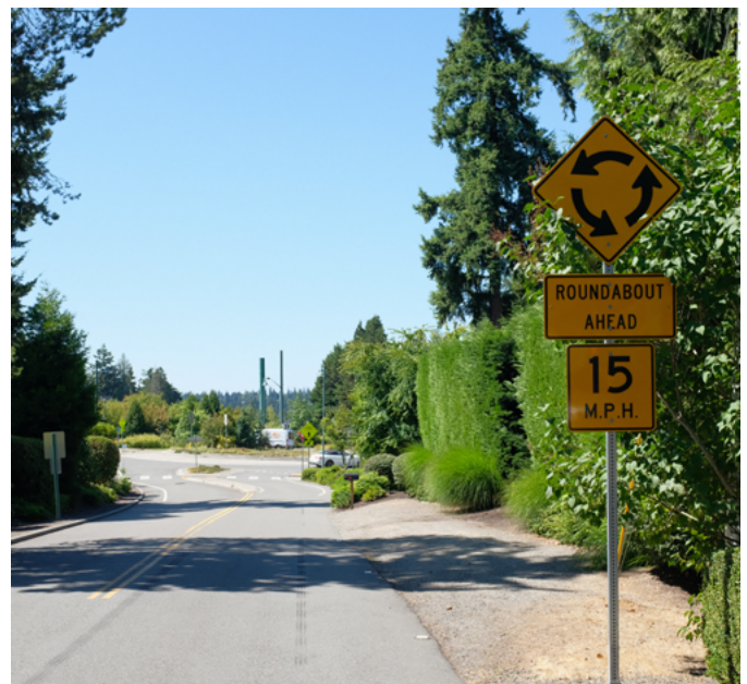
Figure 45. The roundabout (SBN, 2024)
