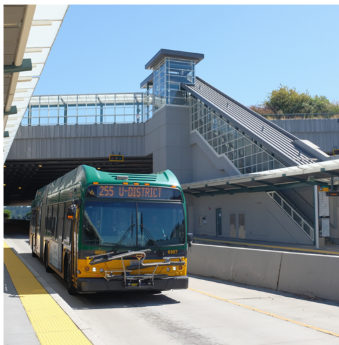
Figure 32. King County Metro Infrastructure (Smith, 2023)
