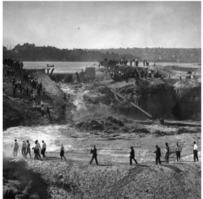
Figure 9. Montelake Cut (MOHAI, 1916)
