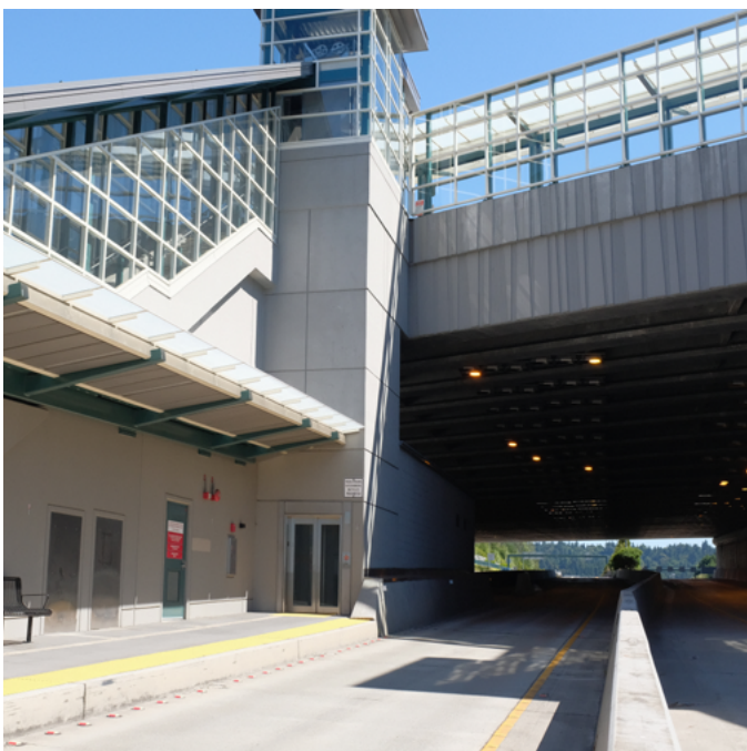
Figure 33. King County Metro Infrastructure (Smith, 2023)
