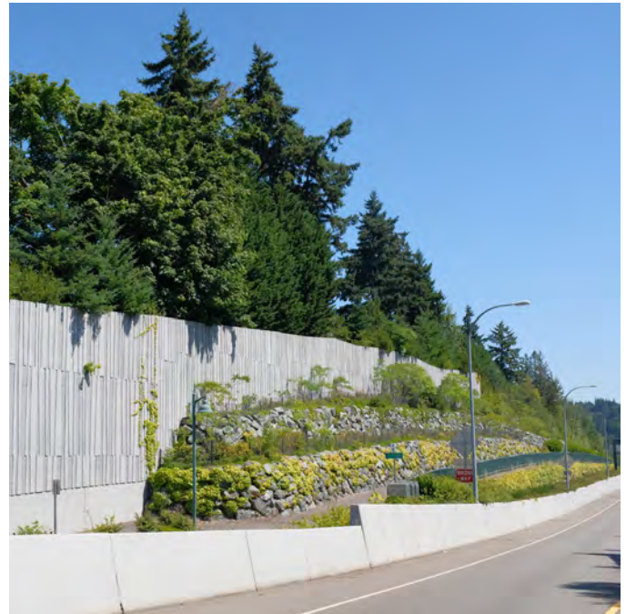
Figure 39. Ramp Barrier Toward SR-520 (Smith, 2023)
