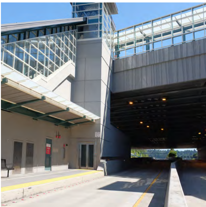
Figure 33. King County Metro Infrastructure (Smith, 2023)
