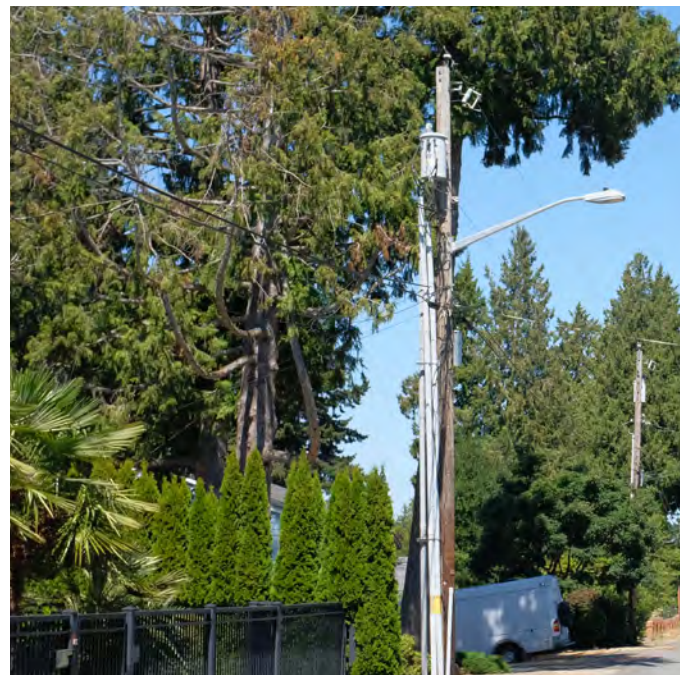
Figure 74. Utility Pole (Smith, 2023)
