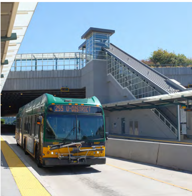
Figure 32. King County Metro Infrastructure (Smith, 2023)
