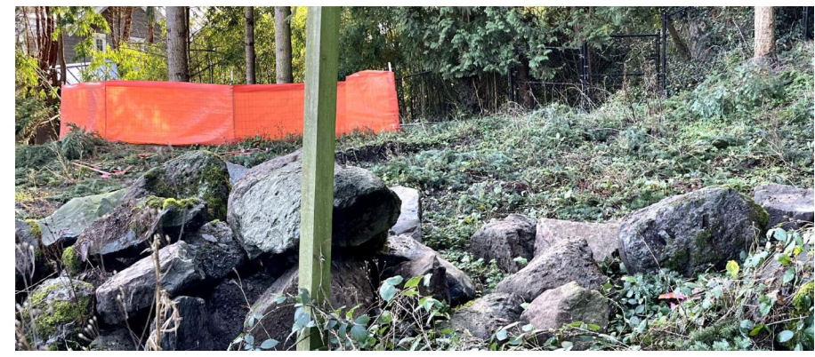
EXISTING ROCKS IN SALLY'S ALLEY PICTURE TAKEN FROM DRIVEWAY AT APPROX. STA. 205+00 LOOKING SOUTHEAST
